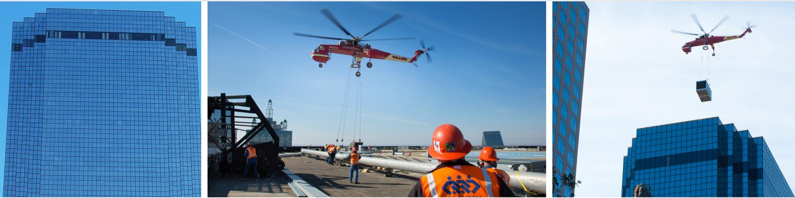
Equipment sizes included (1) 990 ton chiller, (2) 855 ton chillers, (8) 250 ton cooling tower cells, and (96) 10,600 Cubic Feet per Minute (CFM) AHUs with Variable Frequency Drives (VFDs). TD's ability to prefabricate nearly all the piping for the chiller and cooling tower replacements was critical to keeping the project on schedule.
