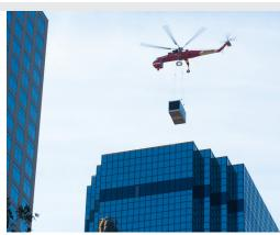
Equipment sizes included (1) 990 ton chiller, (2) 855 ton chillers, (8) 250 ton cooling tower cells, and (96) 10,600 Cubic Feet per Minute (CFM) AHUs with Variable Frequency Drives (VFDs). TD's ability to prefabricate nearly all the piping for the chiller and cooling tower replacements was critical to keeping the project on schedule.
