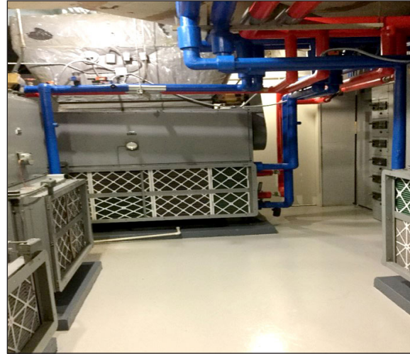
3100 Main, before and after TD's facility maintenance began
